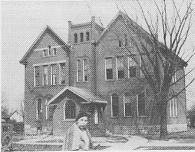
The Harding building, original Grandview Heights school building built in 1895. A similar photo today would show the kindergarten. Courtesy Clarence Salzgeber
