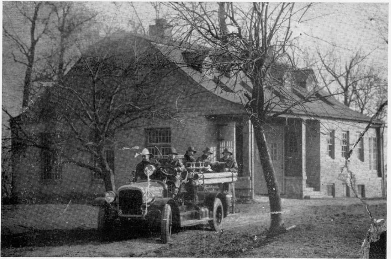
The first fire truck, manned by volunteers, is shown leaving the recently completed Municipal building in 1924. Courtesy Mayor A. K. Pierce
